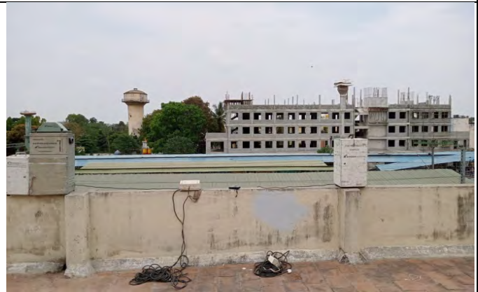
AAQ 4 Yeshwantpur Rly. station
